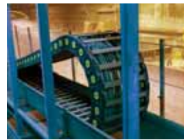
Nylon sliding chains type M80 installed on waste incineration plant "Vestforbrænding" in Denmark
